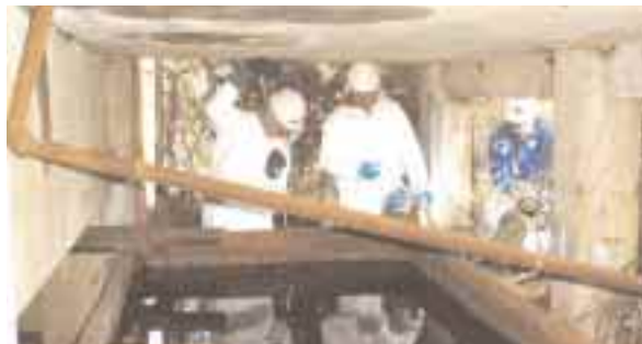
Triad site assessment method leads to discovery of groundwater contamination source, an unsecured vat containing dichlorobenzene (photo by Jeong Seop Shim) at a Brownfield Redevelopment Site. Several days of intensive groundwater testing (50 grab samples from 40 locations) led investigators to the source of dichlorobenzene contamination. Sampling conducted by S2C2, Inc.
