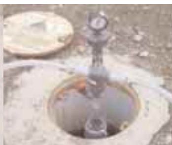
Sulfuric acid injection in progress
