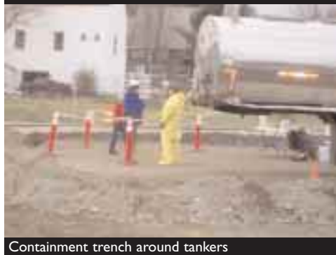
Containment trench around tankers
